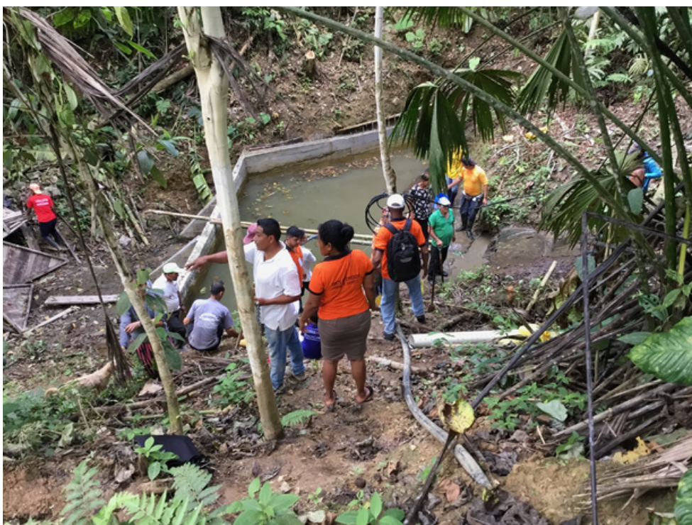
Viche, Esmeraldas Fair Trade USA farmer group aqueduct project construction.
