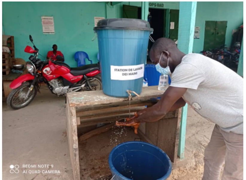
A HAND-WASHING STATION INSTALLED AT A COOP IN IVORY COAST
